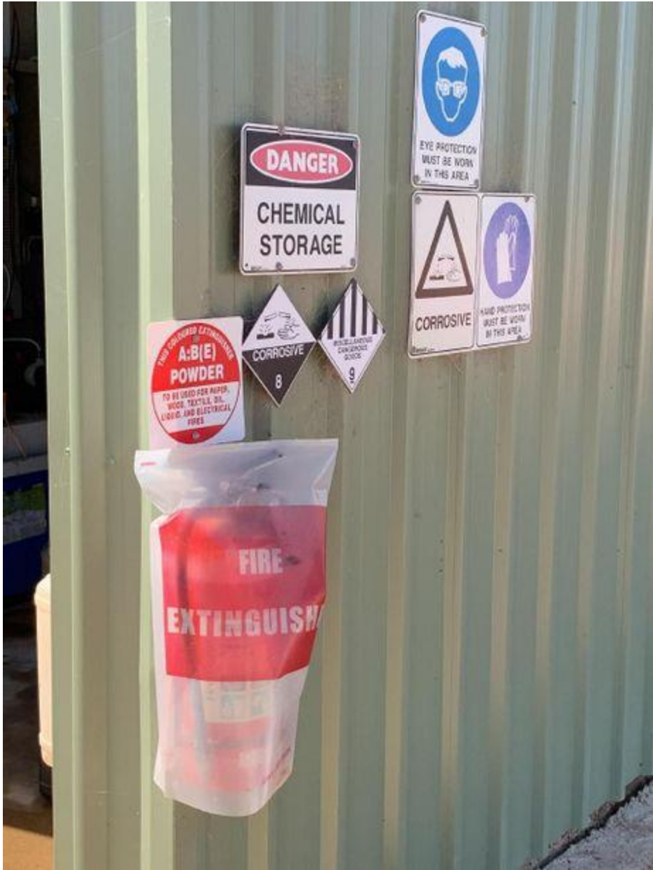
Farm 79 – Safety signage and fire protection on chemical storage shed
