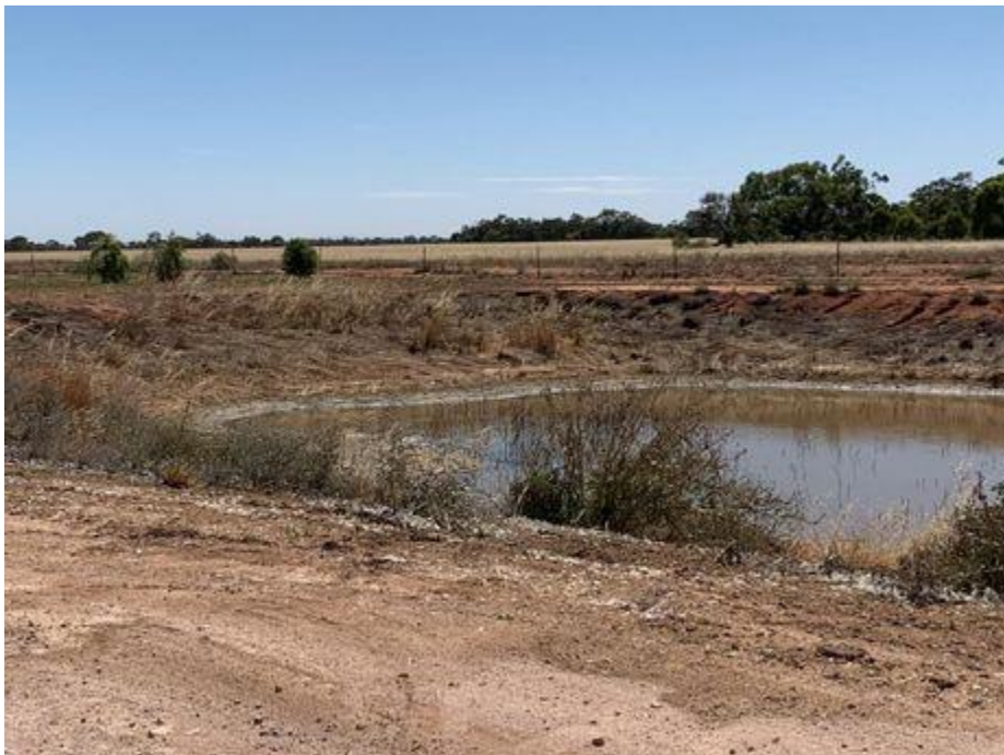
Farm 78 – Sediment basin near empty with signs of erosion in background of photo.
