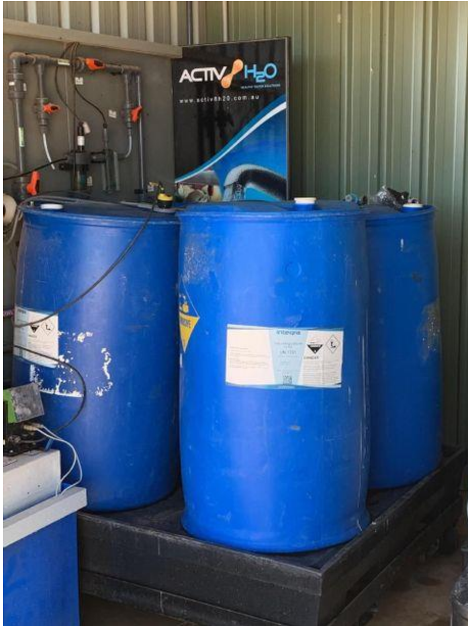
Farm 79 - Chlorine drums on banded pallet in chemical storage shed. Bunded is overloaded with chemical drums too close to the edge of the bund.
