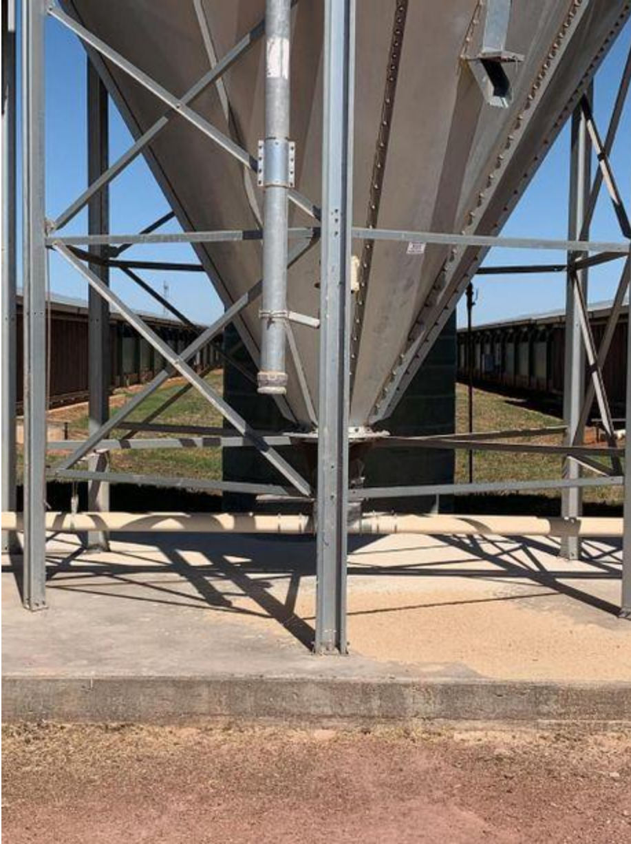
Farm 79 - Spill of feed under silo while in process of setting up sheds.
