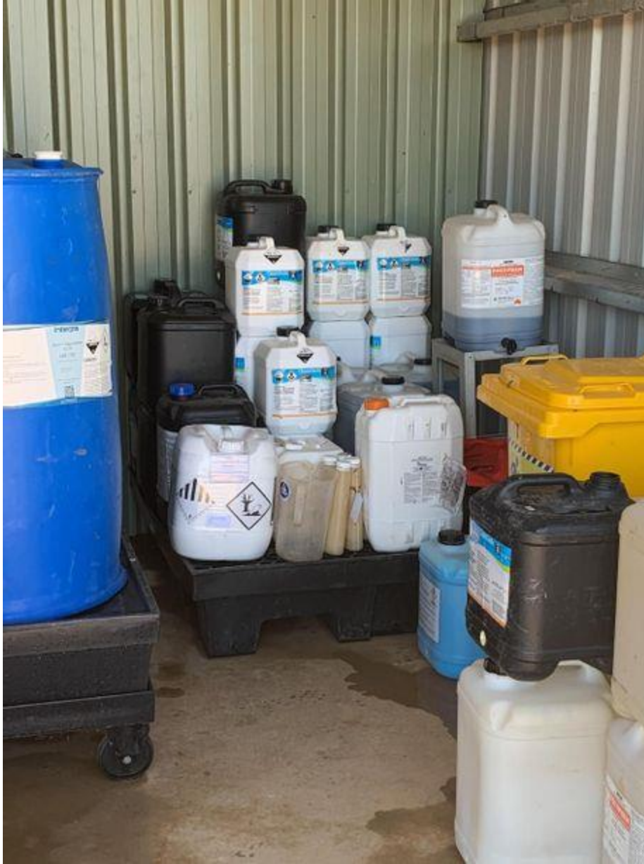
Farm 79 - Other water treatment chemicals on banded pallet in chemical storage shed. Spill kit in yellow bin. Red safety gloves next to spill kit. Evidence of spills on ground. Bund is overloaded with drums too close to the edge of the bund and stacked three high in places.
