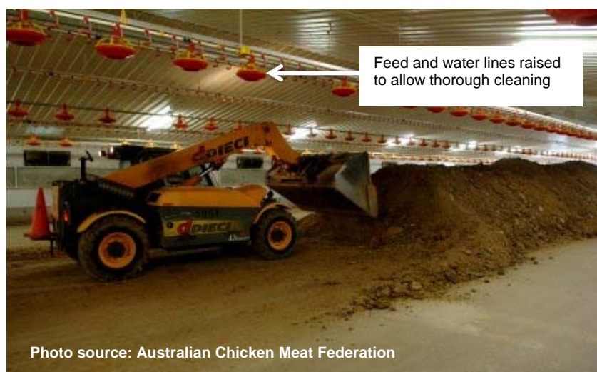
Plate 1 - Poultry Litter Being Removed Using a Front-End Loader
