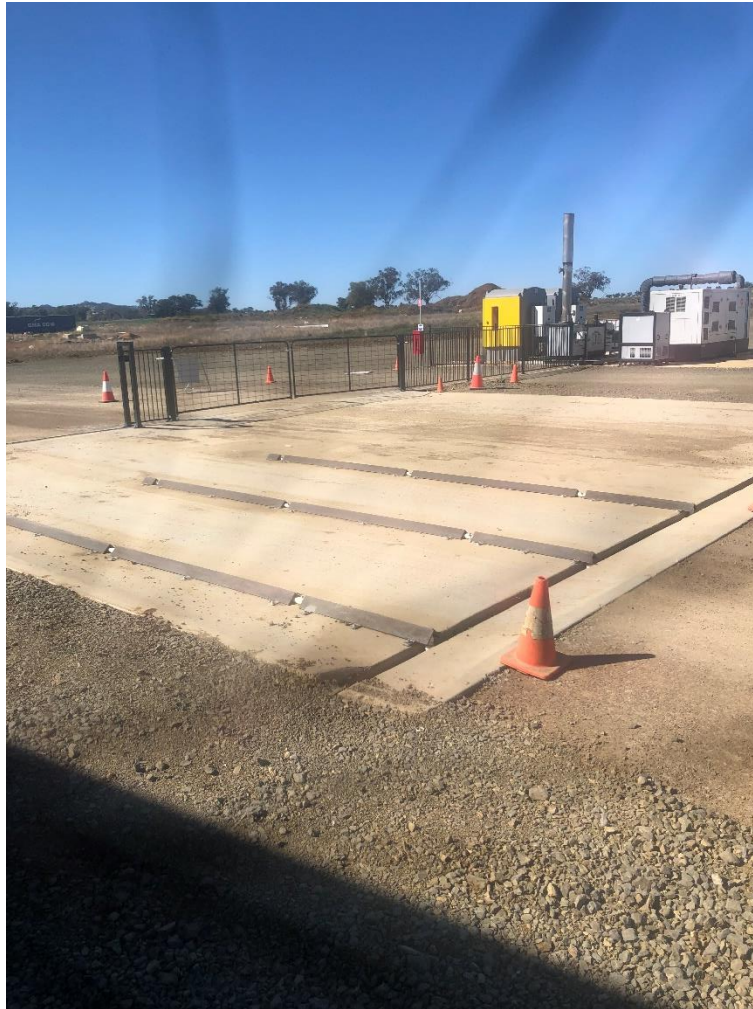
Photo 3 Wheel wash (not operational)
