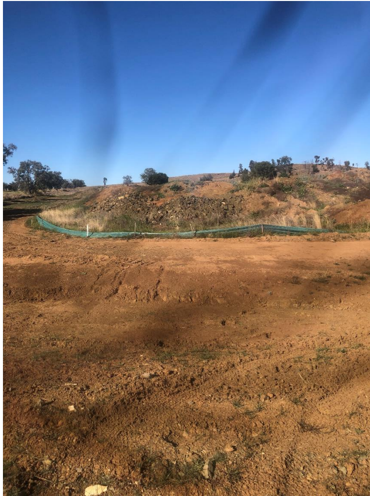
Photo 15 Sediment fencing below the north borrow pit
