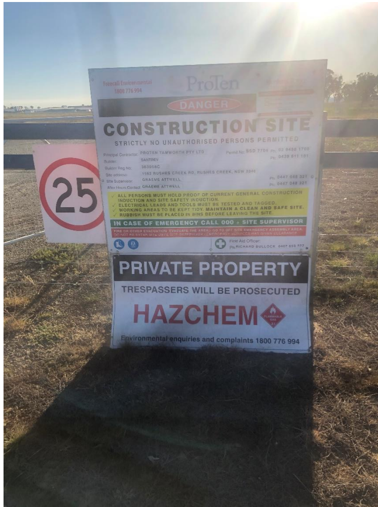
Photo 1 Construction signage at the site entrance
