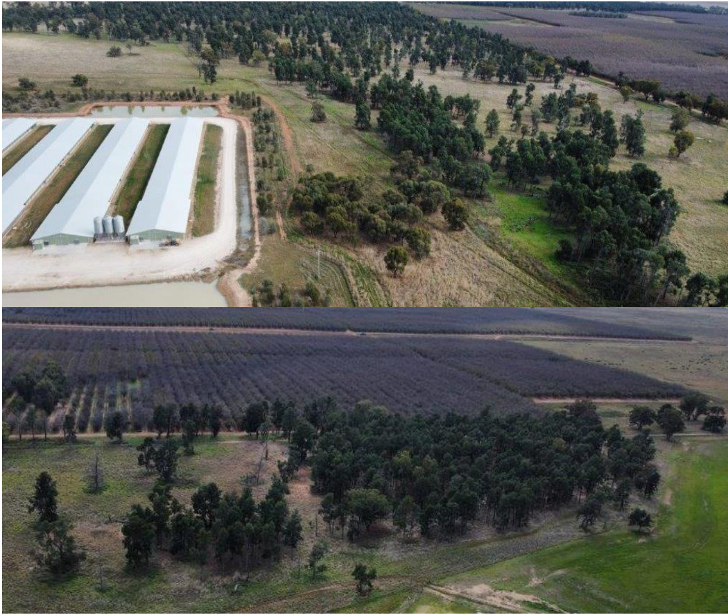
Photo 1 Temporary Offset Area
