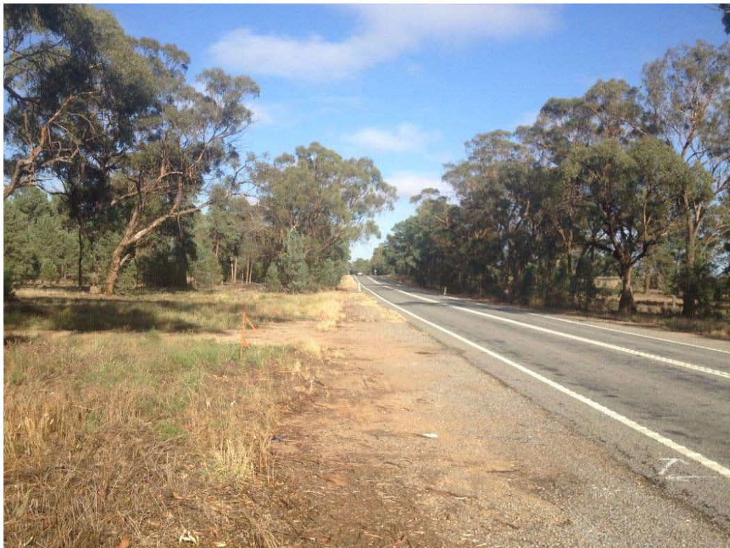
Figure 2.3: Proposed intersection location, looking west towards Darlington Point.
