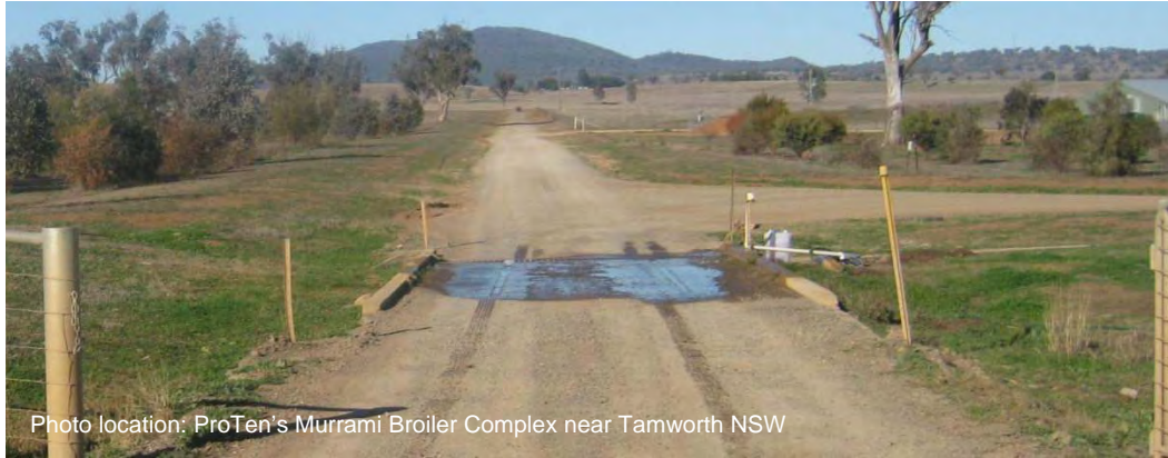
Plate 11 – Example of a wheel wash to be constructed at the farm entrance
