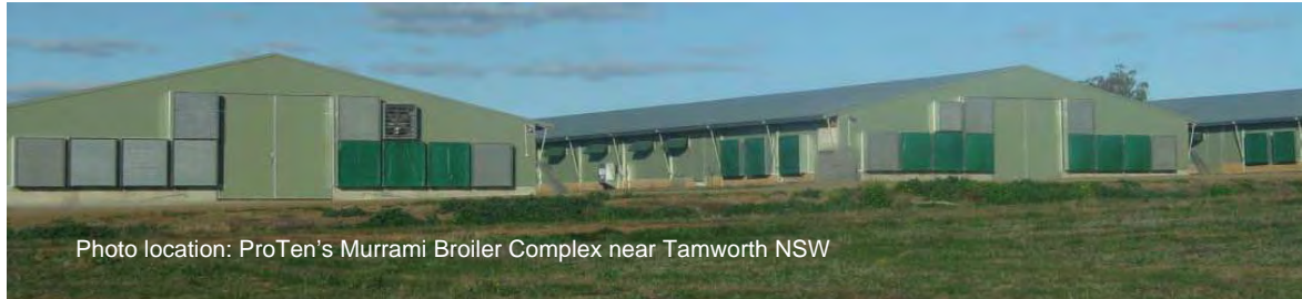
Plate 5 – Broiler Shed Exhaust Fans
