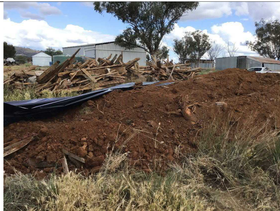
Photograph 10 – Stockpiled material from unexpected finds, facing east
