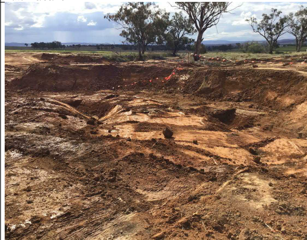
Photograph 16 – Adjacent TP303 facing west, post excavation
