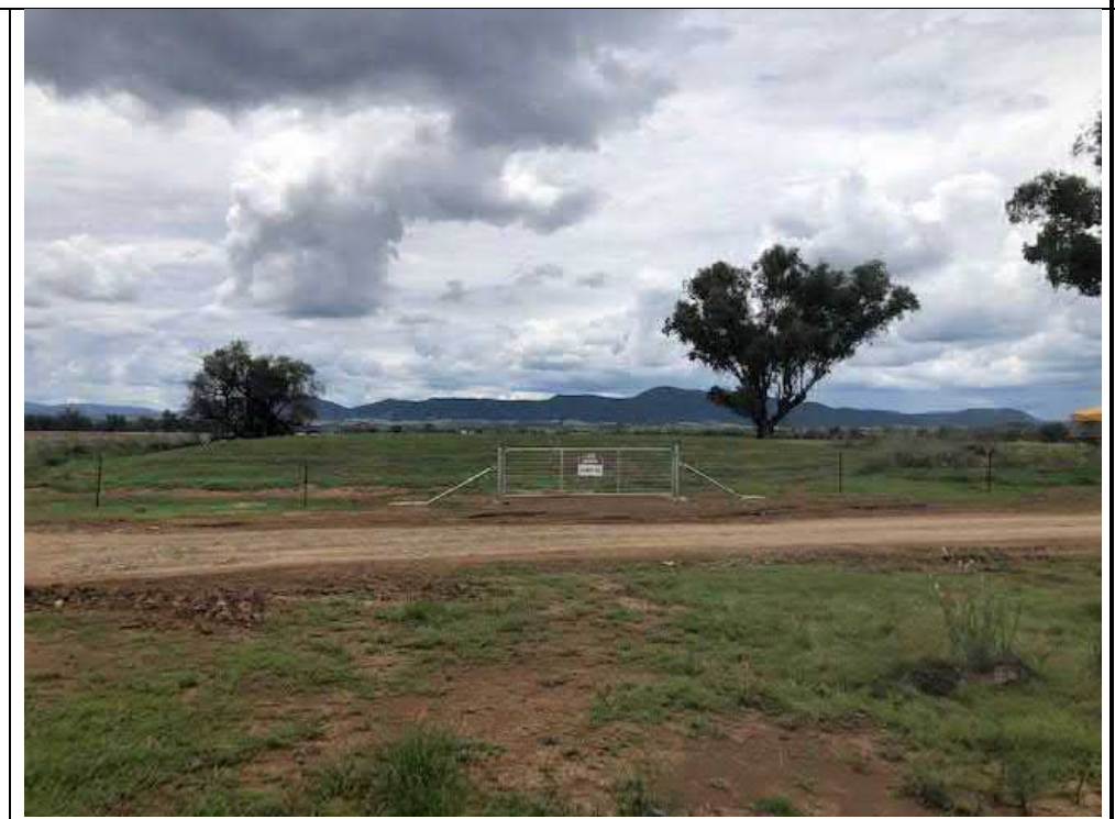
Photograph 35 – Capping area showing fencing and revegetation
