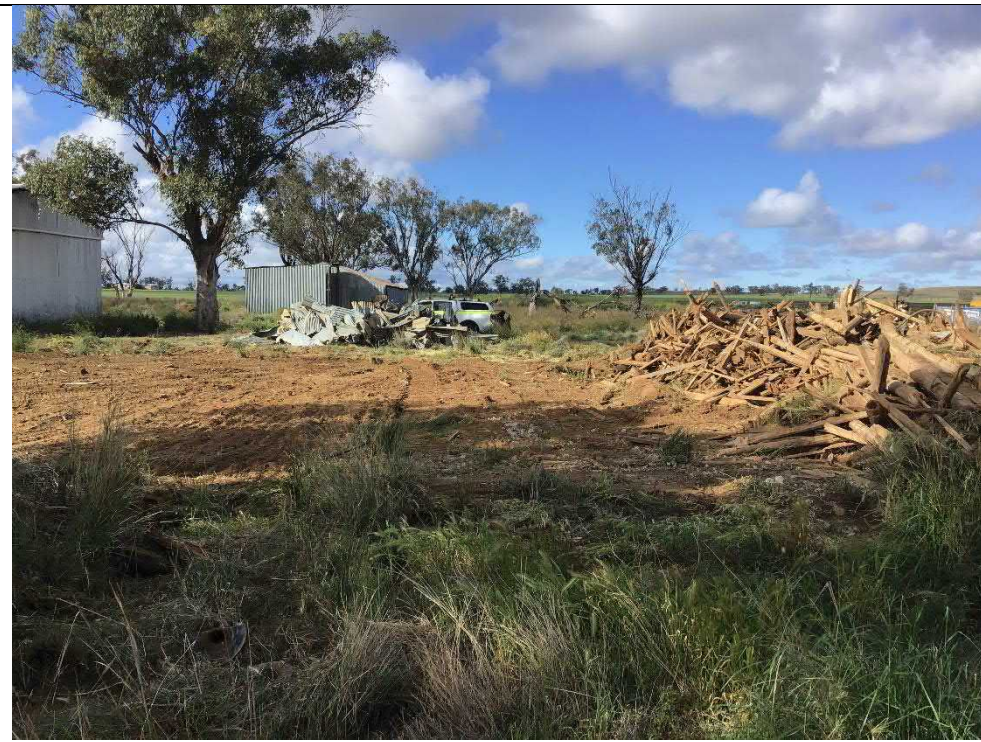
Photograph 3 – Capping area prior to remediation facing south from TP205, showing stockpiled timber from former sheep shed
