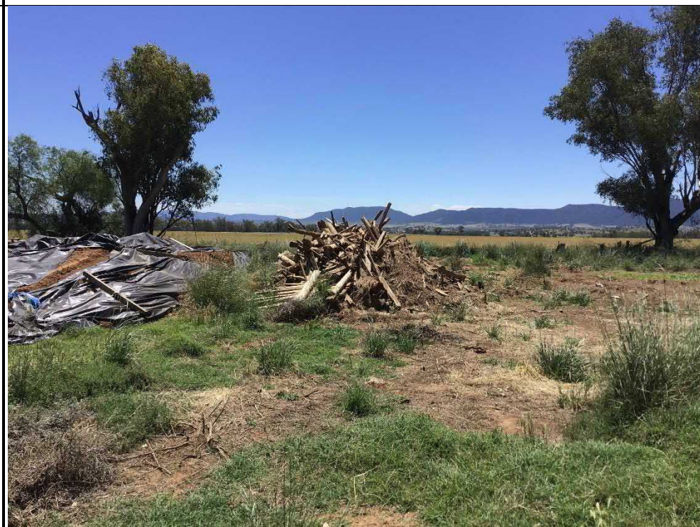
Photograph 19 – Timber Stockpile from demolition of sheep holding shed, facing north from TP201
