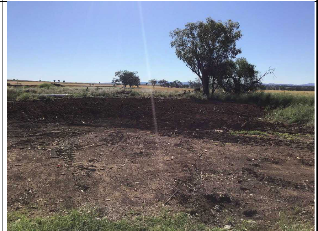
Photograph 24 – Unexpected finds stockpile spread within the remediation area to form part of the Earth Cover Layer of capping, from adjacent TP103
