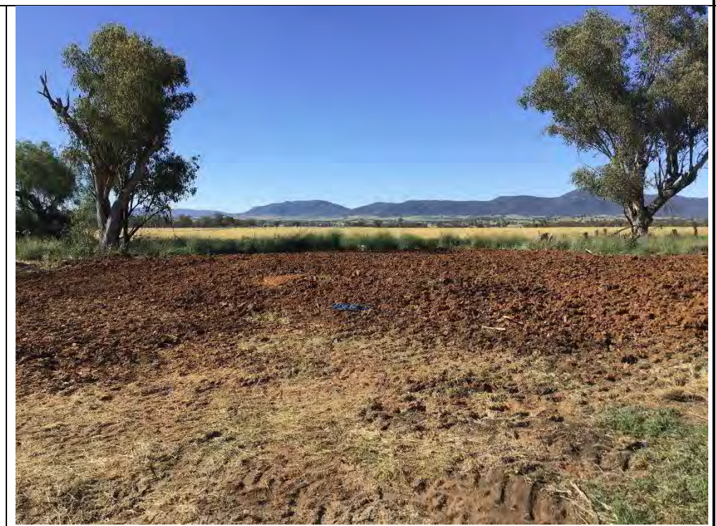
Photograph 23 – Unexpected finds stockpile spread within the remediation area to form part of the Earth Cover Layer of capping, from TP201
