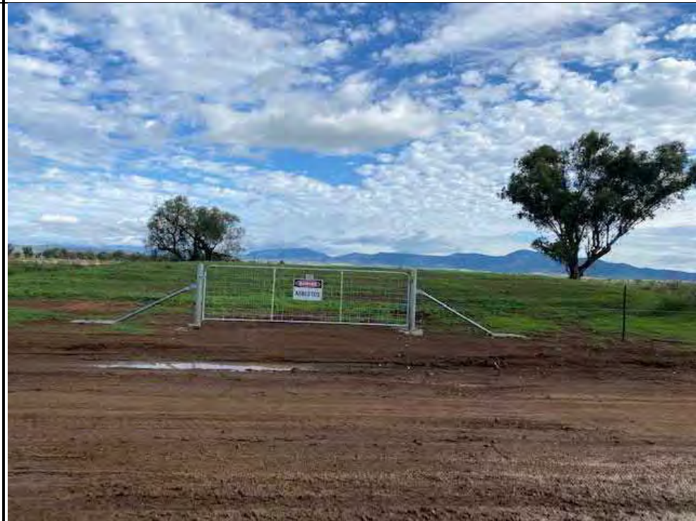
Photograph 38 - Capping area showing fencing with asbestos signage and revegetation
