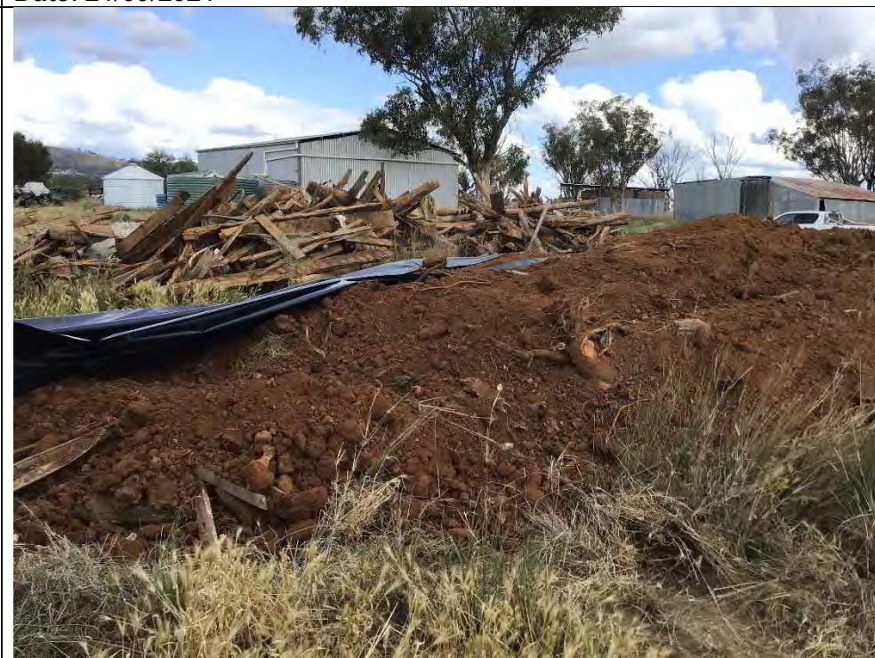
Photograph 10 – Stockpiled material from unexpected finds, facing east
