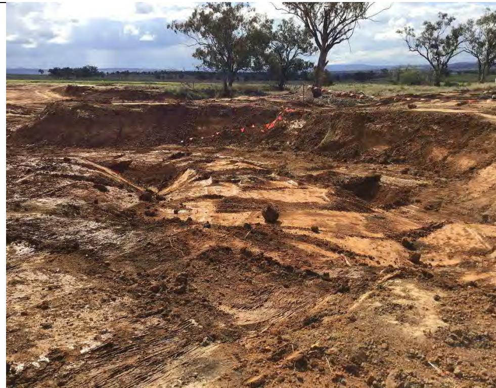
Photograph 16 – Adjacent TP303 facing west, post excavation
