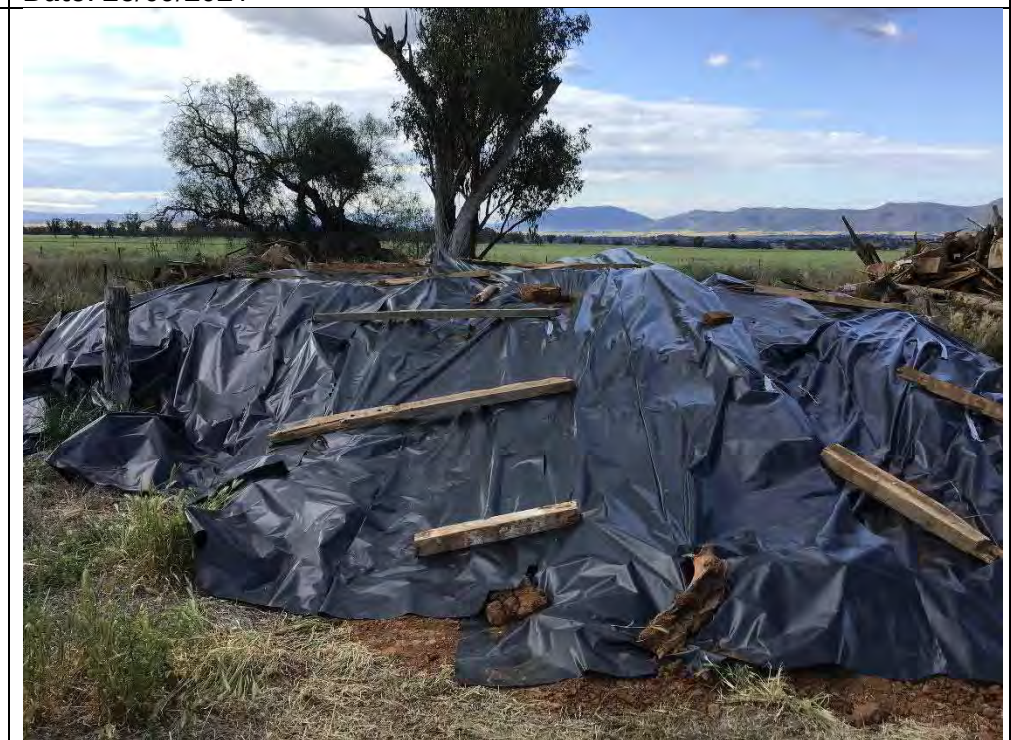
Photograph 12 – Covered stockpile of unexpected find material, facing north from between TP201 and TP202
