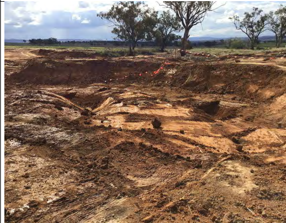
Photograph 16 – Adjacent TP303 facing west, post excavation
