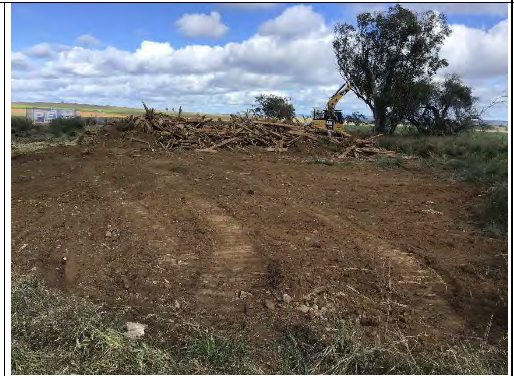
Photograph 5 Capping area prior to remediation facing west from TP103
