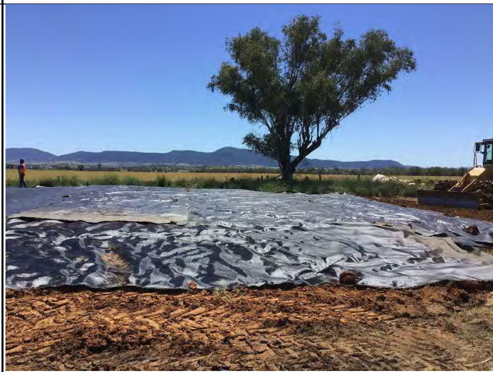
Photograph 25 – Marker layer over Earth Cover Layer, facing north from adjacent TP201
