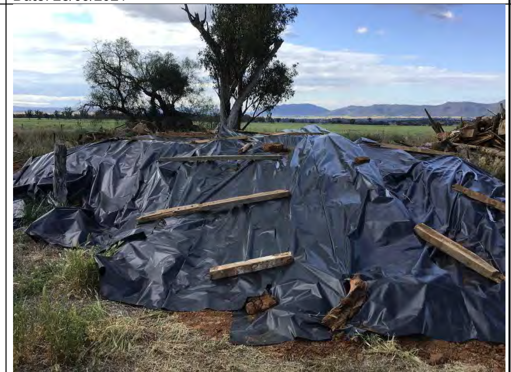
Photograph 12 – Covered stockpile of unexpected find material, facing north from between TP201 and TP202
