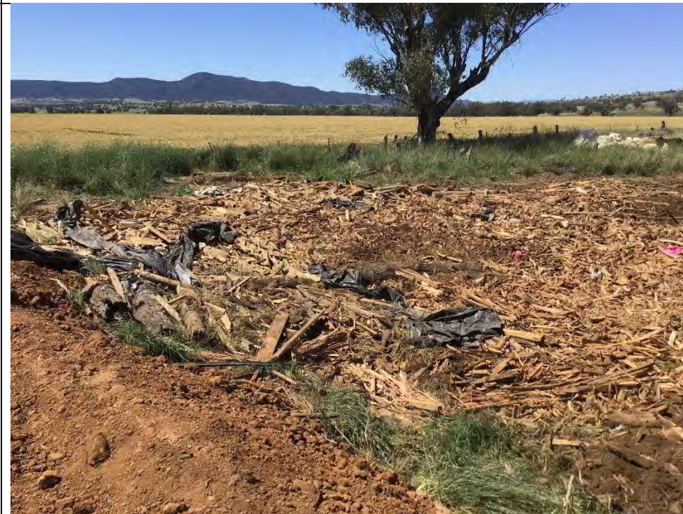
Photograph 22 – Timber stockpile spread and compacted into surface within the remediation area, facing north from adjacent TP202
