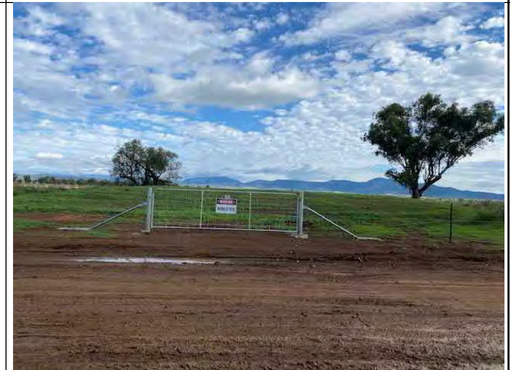
Photograph 36 – Capping area showing fencing with asbestos signage and revegetation
