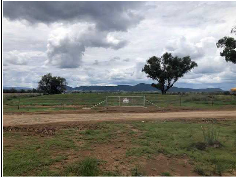
Photograph 37 – Capping area showing fencing and revegetation
