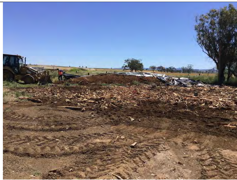
Photograph 21 – Timber stockpile spread and compacted into surface within the remediation area, from adjacent TP 103
