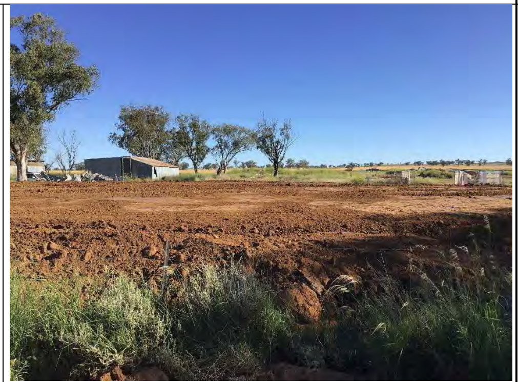
Photograph 35 – Topsoil layer, facing south
