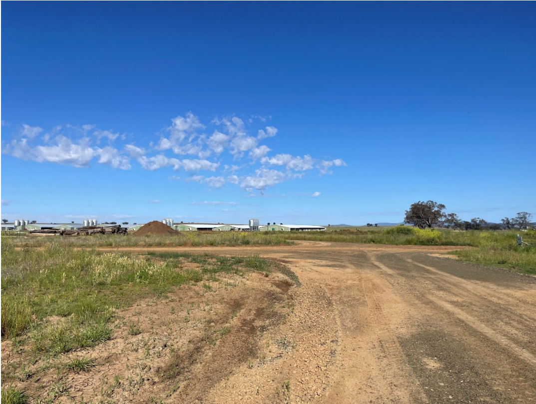
Photo 6: Internal roads – some require reapplication of gravel to minimise dust.
