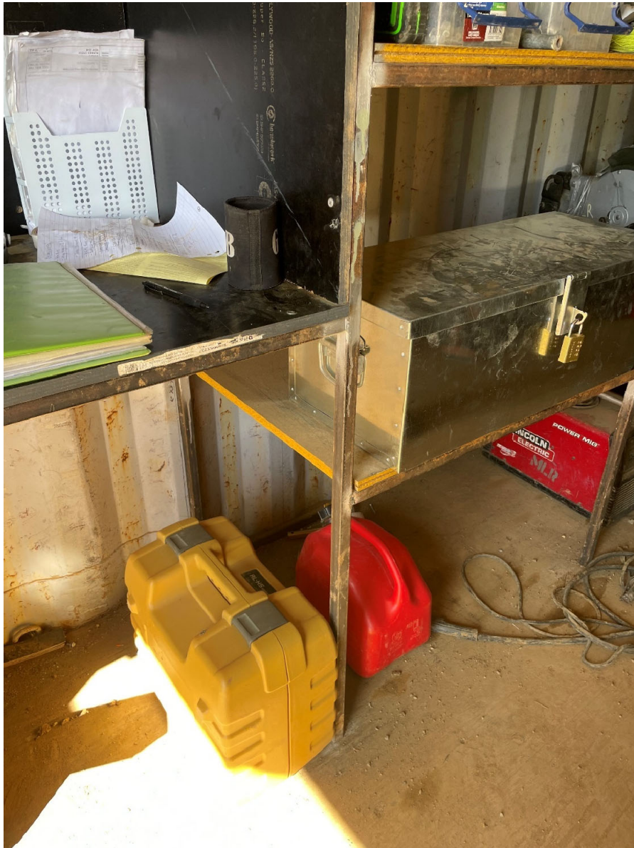
Photo 24: Inside shipping container used for storage during construction. Small fuel container on floor of container presents a risk of minor spills. It is noted appropriate bunds are present and in use inside the amenities/office shed of Farm 2.
