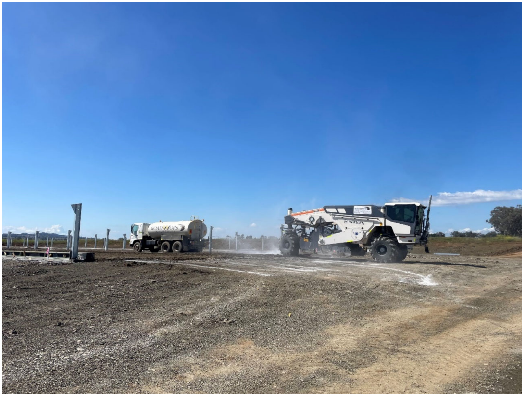
Photo 28: Construction of Shed 18 at Farm 2. Water truck in use.
