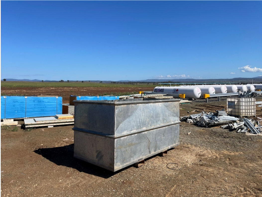
Photo 27: Cleanaway bins and equipment on western side of Farm 2.
