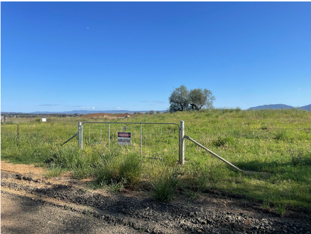
Photo 7: Remediation site fully fenced and capping intact.
