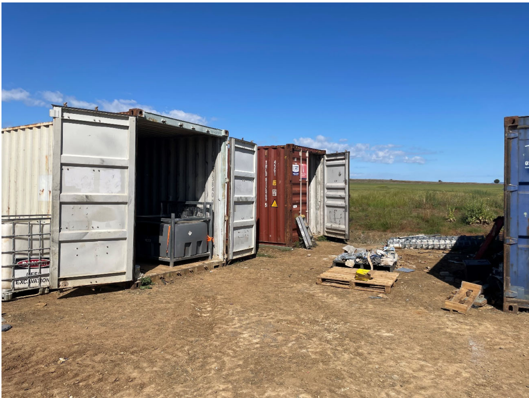
Photo 23: Storage containers for construction.
