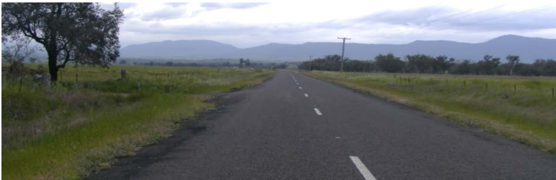
Photo 24 Rushes Creek Road looking northbound adjacent to the Development Site near the existing access in to Lot 165 (on LHS)
