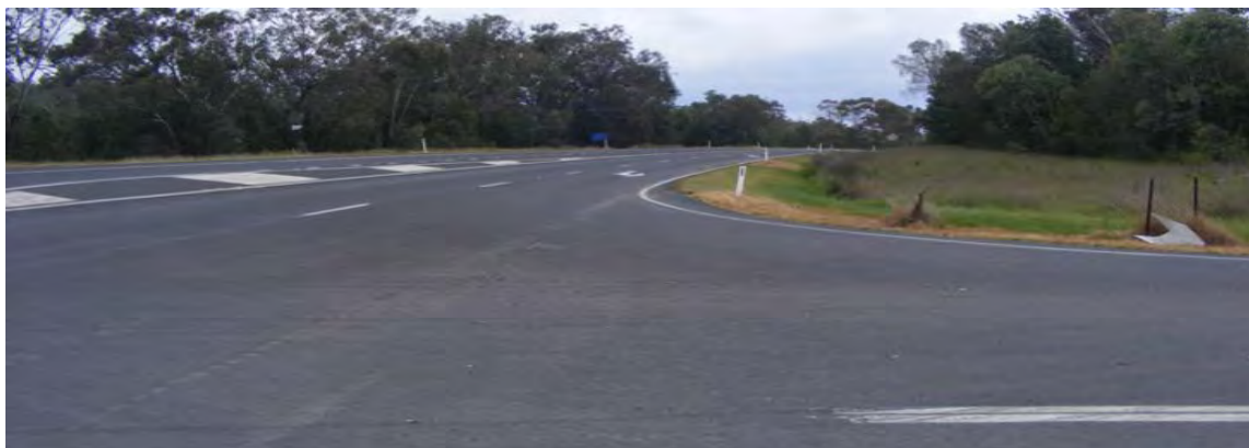
Photo 28 Oxley Highway / Rushes Creek Road intersection looking west
