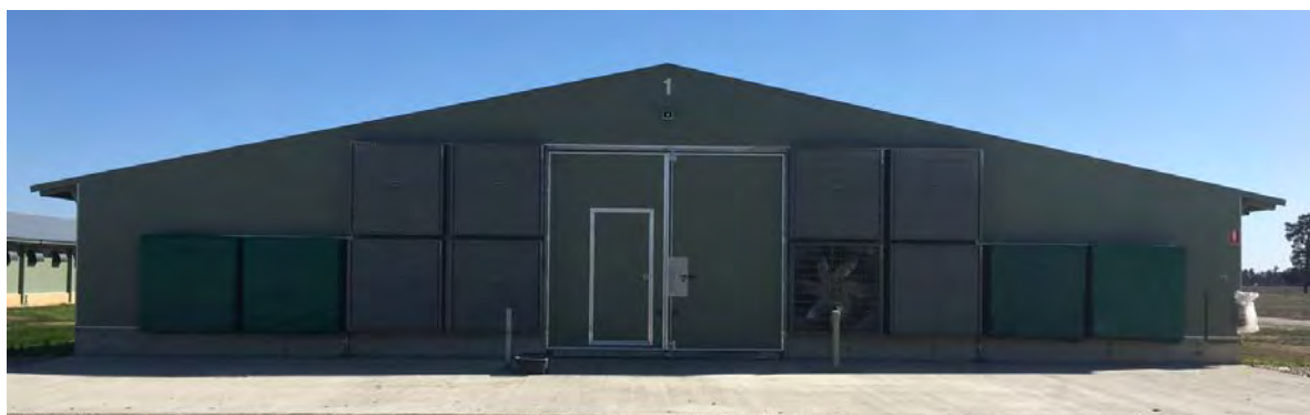
Photo 8 Tunnel ventilation fans (ProTen’s Narrandera Poultry Production Farm)
