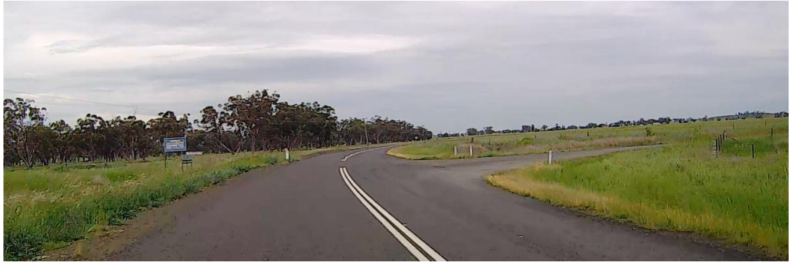
Figure 2.5: Rushes Creek Road looking southbound at Ski Gardens Road
