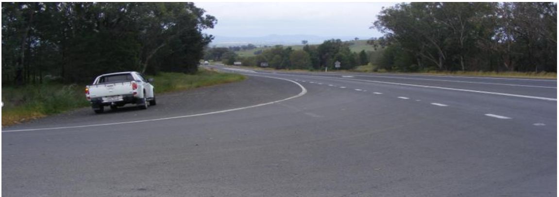
Figure 2.11: Oxley Highway / Rushes Creek Road intersection looking east
