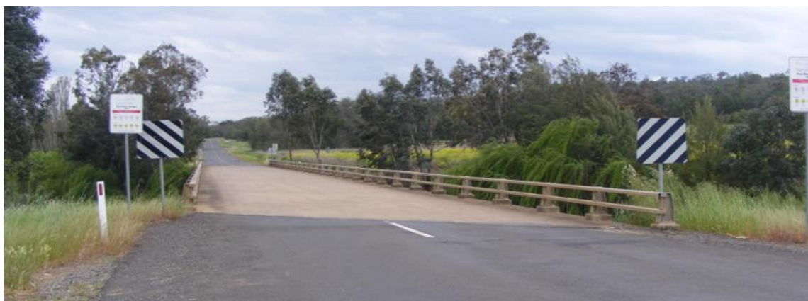
Figure 2.3: Rushes Creek Road looking southbound at Peel River Bridge
