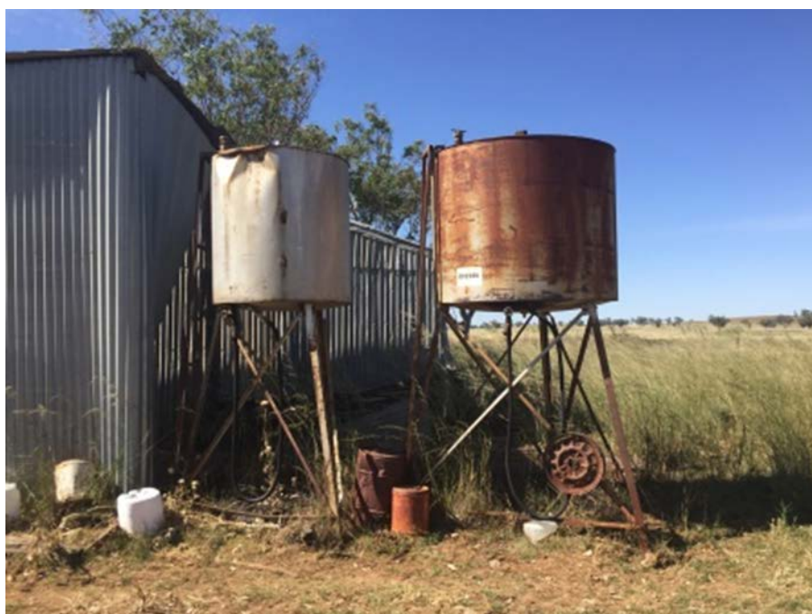
Photo 24 Septic tank in Lot 165
