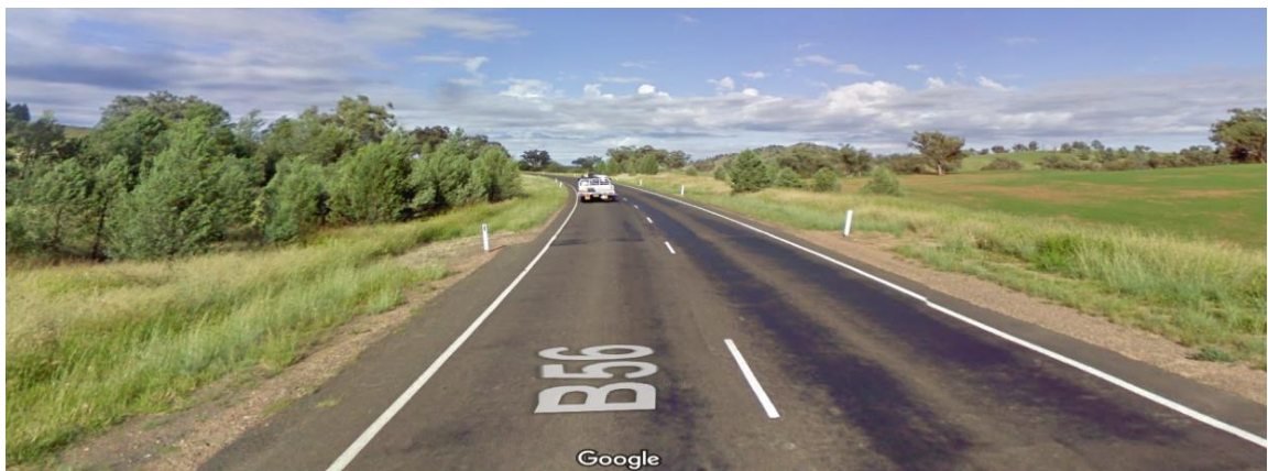
Figure 2.2: Looking west along Oxley Highway to the west of Rushes Creek Road (Source: Google Maps)
