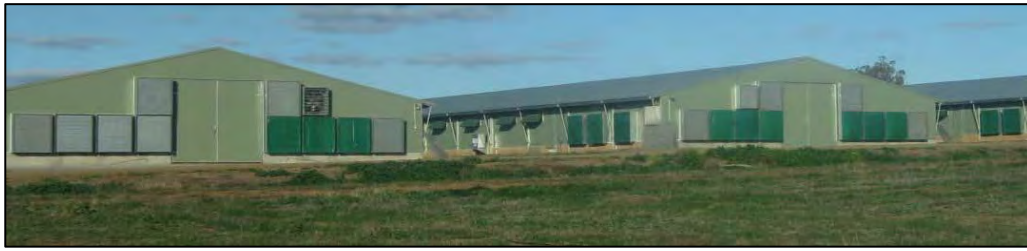
Figure 1-3: Example of poultry sheds from ProTen's Murrami PPUs (Somerton, NSW).
