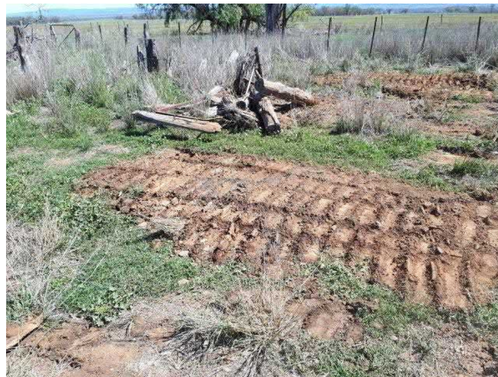
Photograph 5 – Backfilling of test-pit
