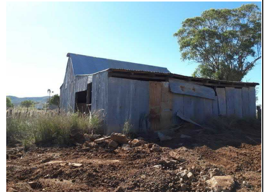
Photograph 12 – View of location of former sheep dip beside sheep holding shed after backfilling
