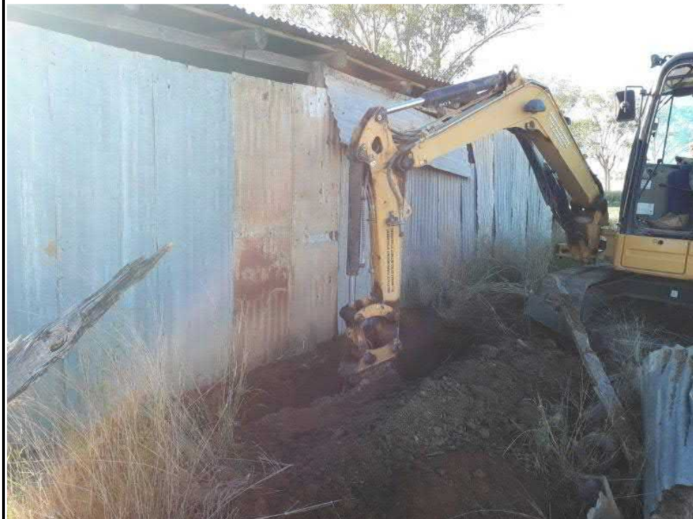
Photograph 10 – Excavator working on test-pit between sheep dip and sheep holding shed
