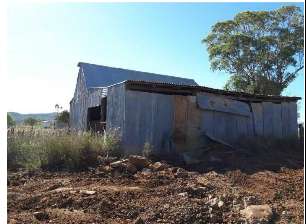
Photograph 12 – View of location of former sheep dip beside sheep holding shed after backfilling
