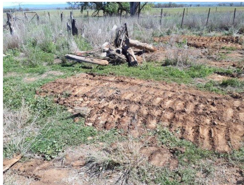
Photograph 5 – Backfilling of test-pit
