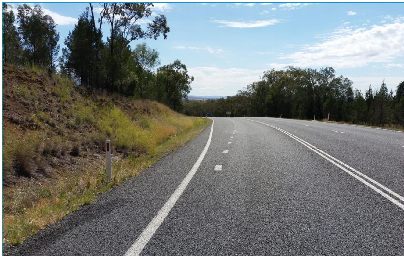
Figure 7 Looking East along the Oxley Highway towards Rushes Creek Road
