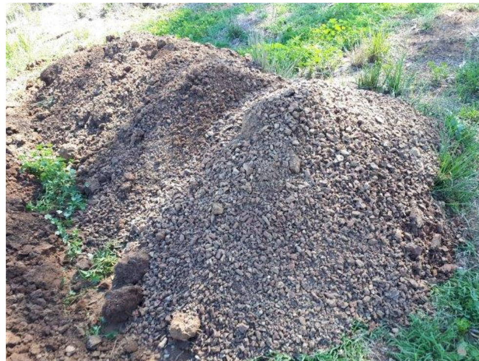
Photograph 11 – Excavated soil from test-pit
