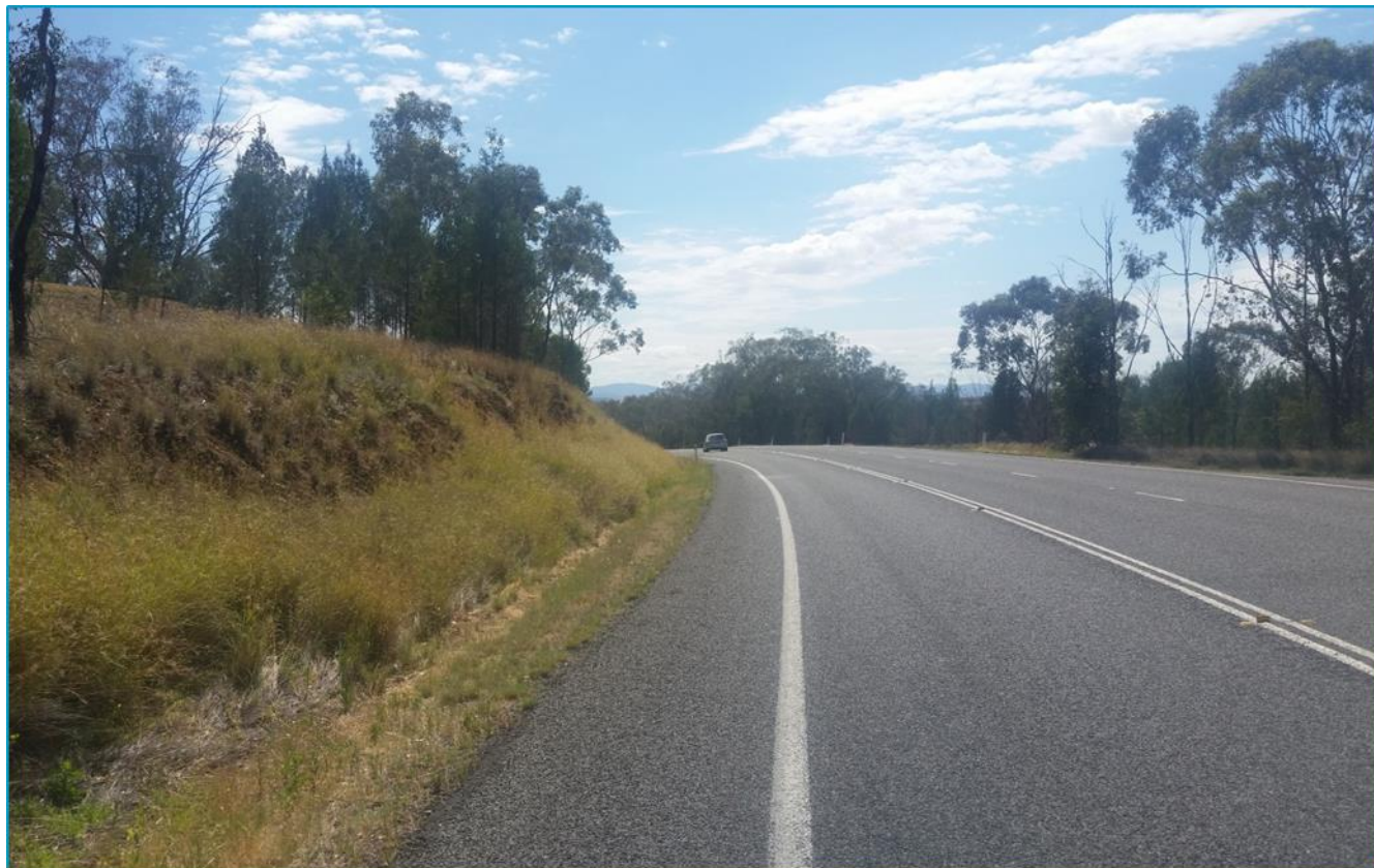
Figure 6 Looking East along the Oxley Highway towards Rushes Creek Road
