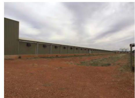
Photograph 3 Poultry Shed No.1 (view of shed length)
