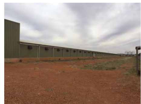
Photograph 3 Poultry Shed No.5 (view of shed length)
