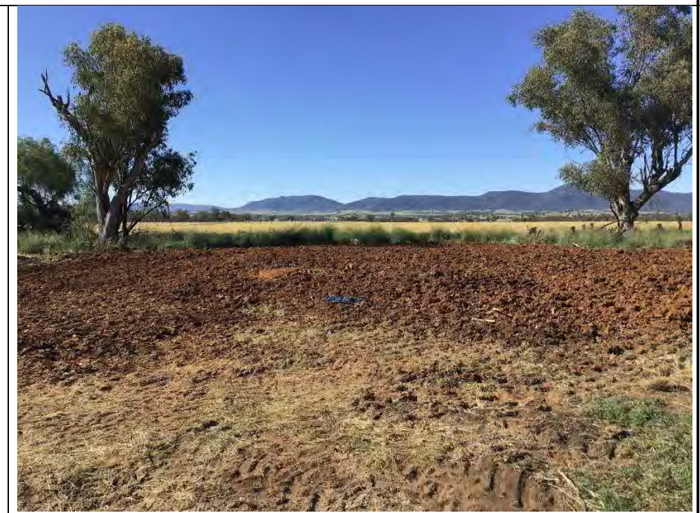
Photograph 23 – Unexpected finds stockpile spread within the remediation area to form part of the Earth Cover Layer of capping, from TP201
