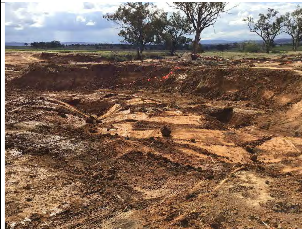
Photograph 16 – Adjacent TP303 facing west, post excavation
