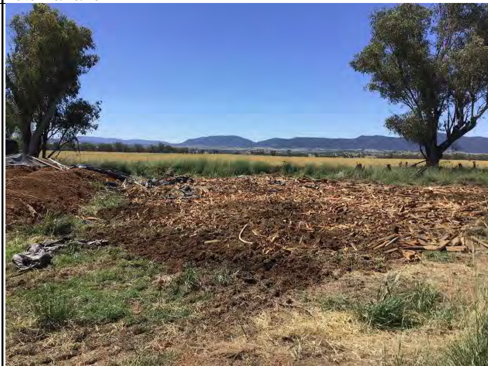
Photograph 20 – Timber stockpile spread and compacted into surface within the remediation area, facing north from TP 201
