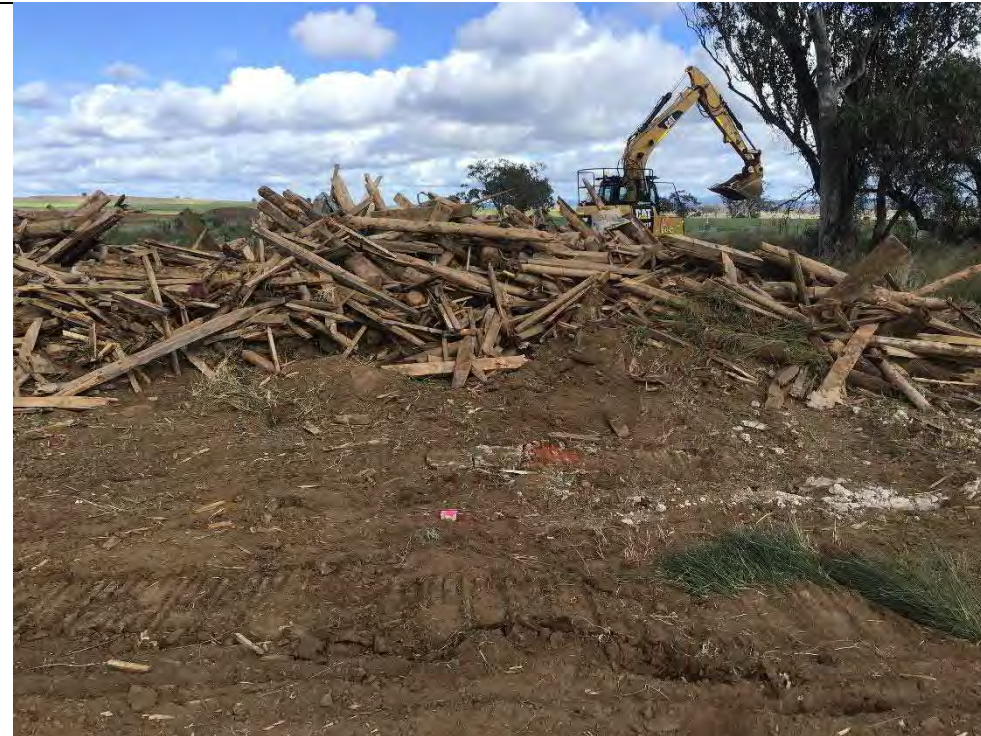
Photograph 4 – Timber stockpile from sheep holding shed demolition, facing west from TP102
