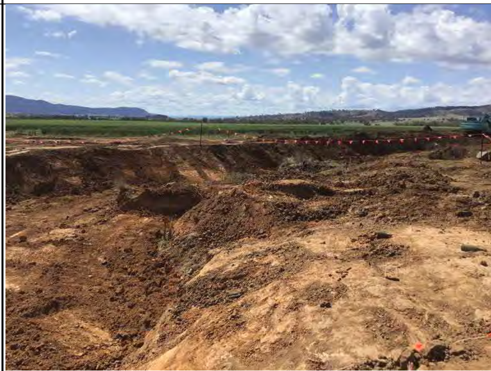
Photograph 13 – TP301 facing east, pre-excitation
