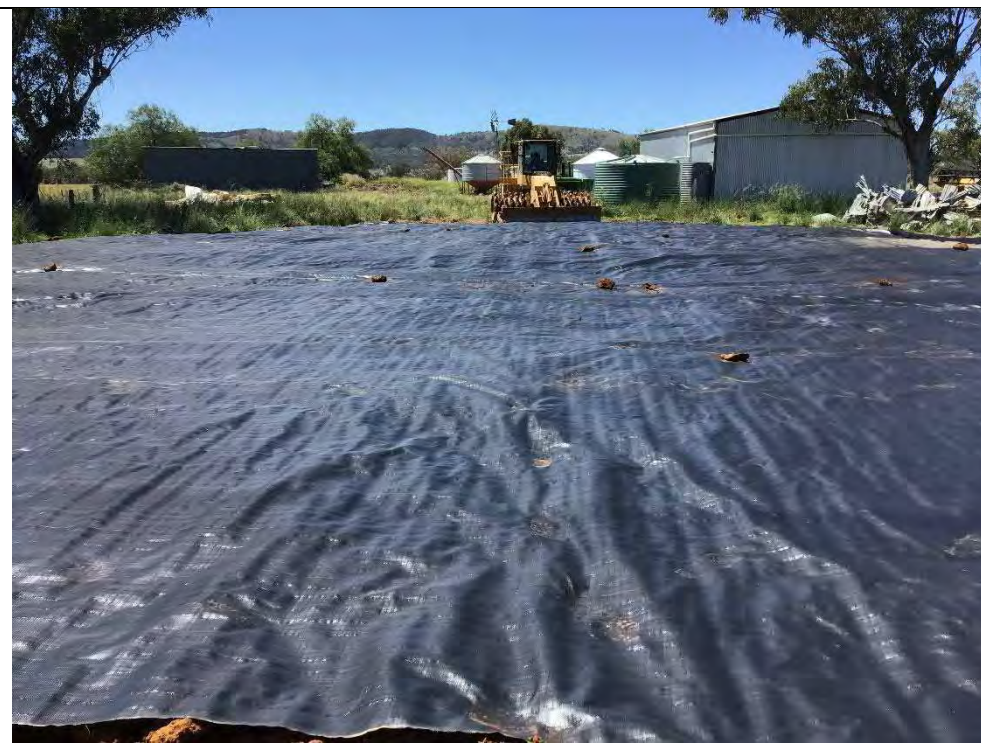
Photograph 27 – Marker layer over Earth Cover Layer, facing east from adjacent TP204
