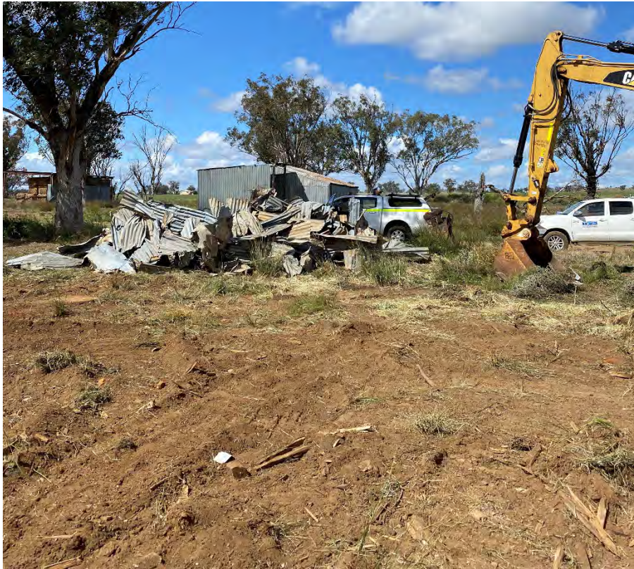
Figure 4 Metal from demolition of shed looking south.
