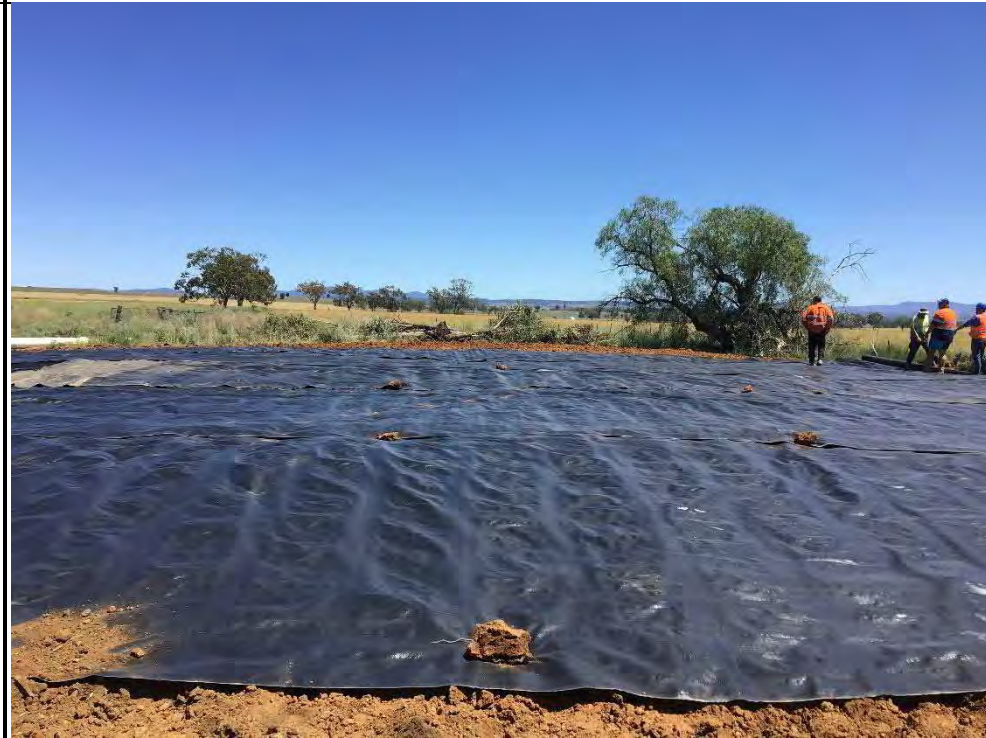
Photograph 26 – Marker layer over Earth Cover Layer, facing west from adjacent TP102
