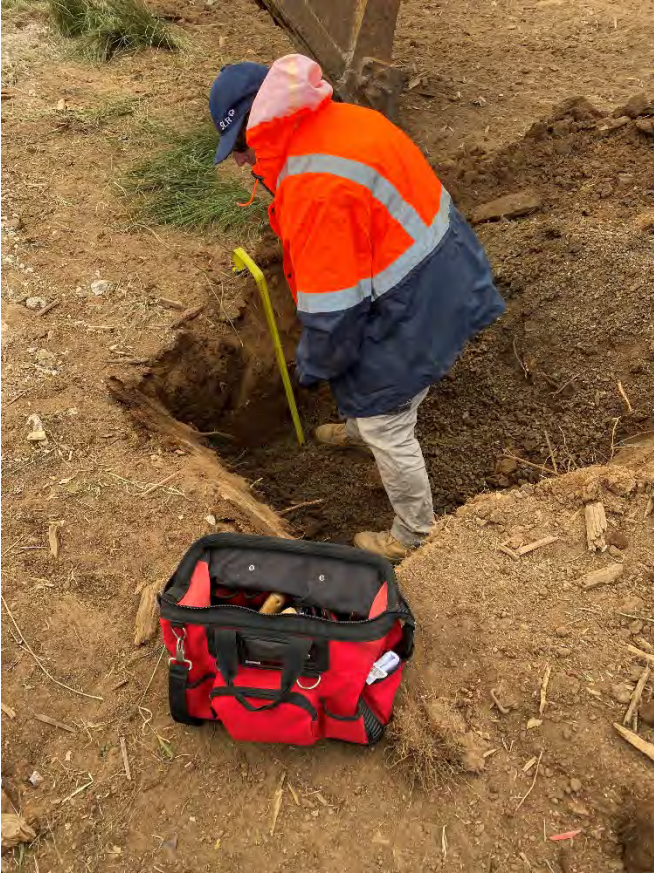
Figure 7 Sampling of test pit TP101
