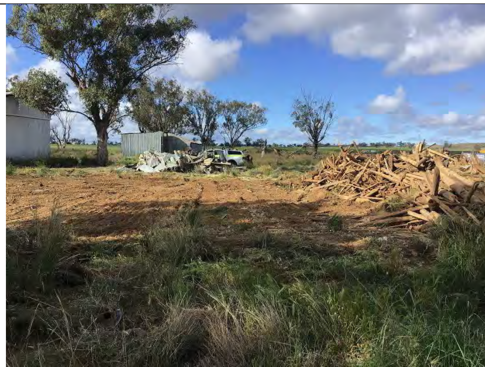
Photograph 3 – Capping area prior to remediation facing south from TP205, showing stockpiled timber from former sheep shed
