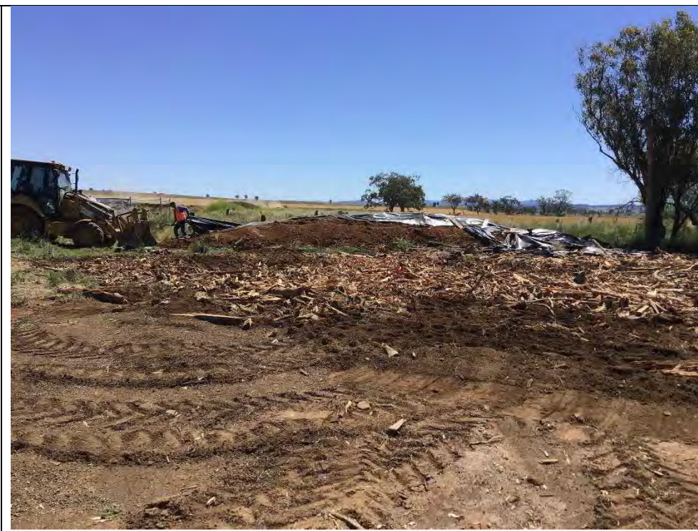
Photograph 21 – Timber stockpile spread and compacted into surface within the remediation area, from adjacent TP 103
