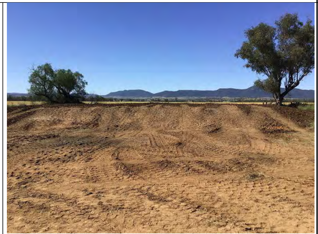
Photograph 29 – Low permeability clay layer, facing north adjacent TP202
