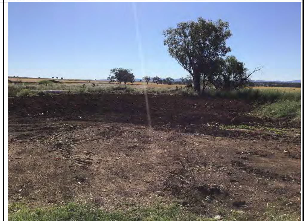
Photograph 24 – Unexpected finds stockpile spread within the remediation area to form part of the Earth Cover Layer of capping, from adjacent TP103
