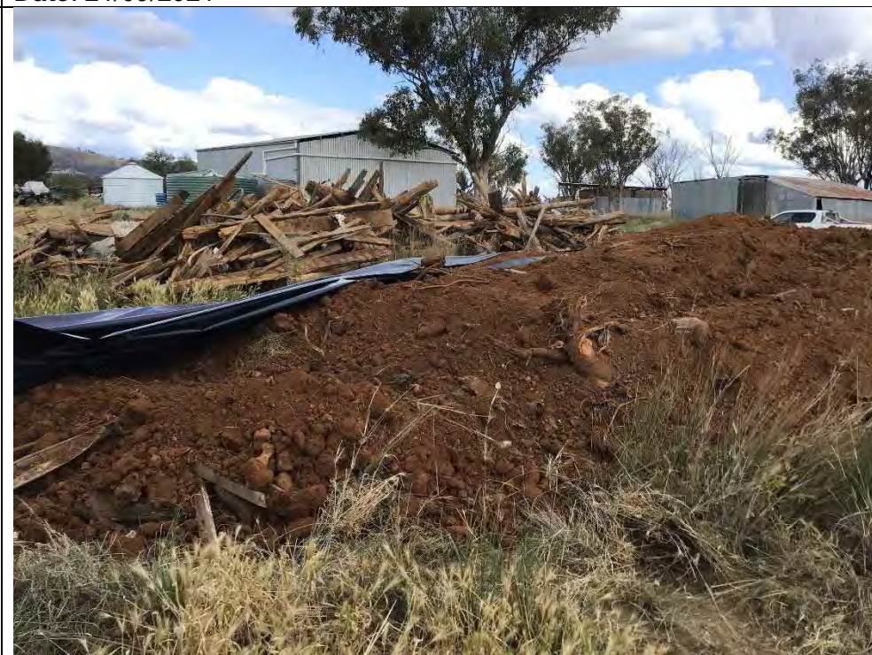
Photograph 10 – Stockpiled material from unexpected finds, facing east
