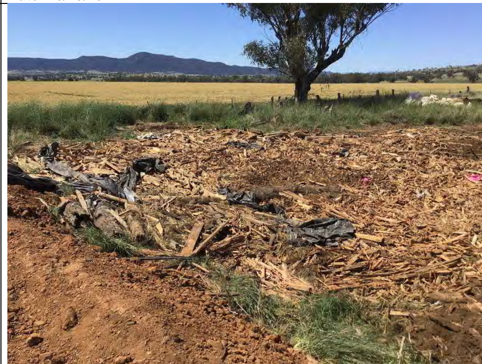
Photograph 22 – Timber stockpile spread and compacted into surface within the remediation area, facing north from adjacent TP202
