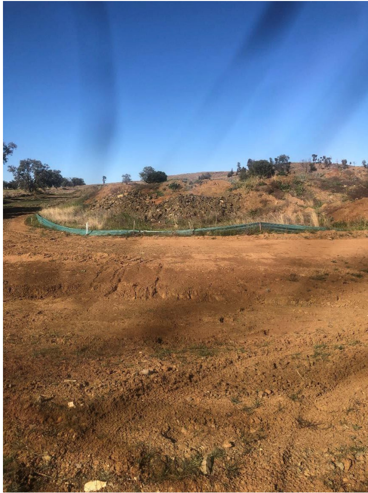
Photo 15 Sediment fencing below the north borrow pit
