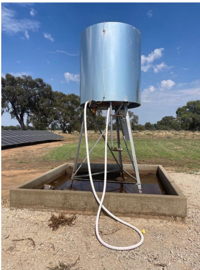
Photo 8 Fuel storage including the screening around the outside to prevent punctures of the tank. Some water inside tank bunds to be pumped out. Hoses should be returned to inside of the bund.
