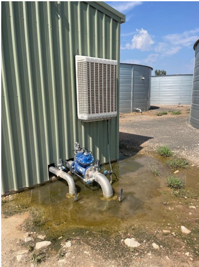
Photo 2 Water leak (untreated water) from water treatment shed.
