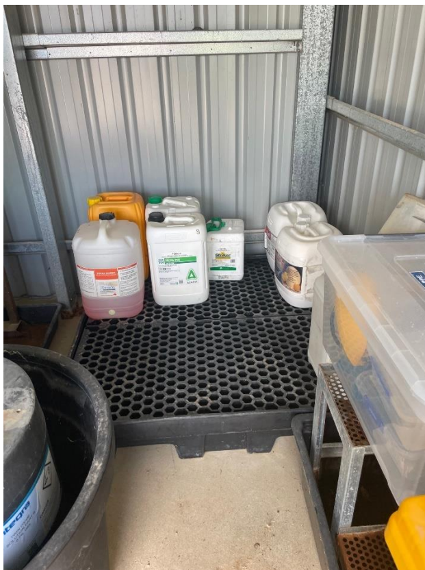
Photo 6 Chemical stored on appropriate bunding.
