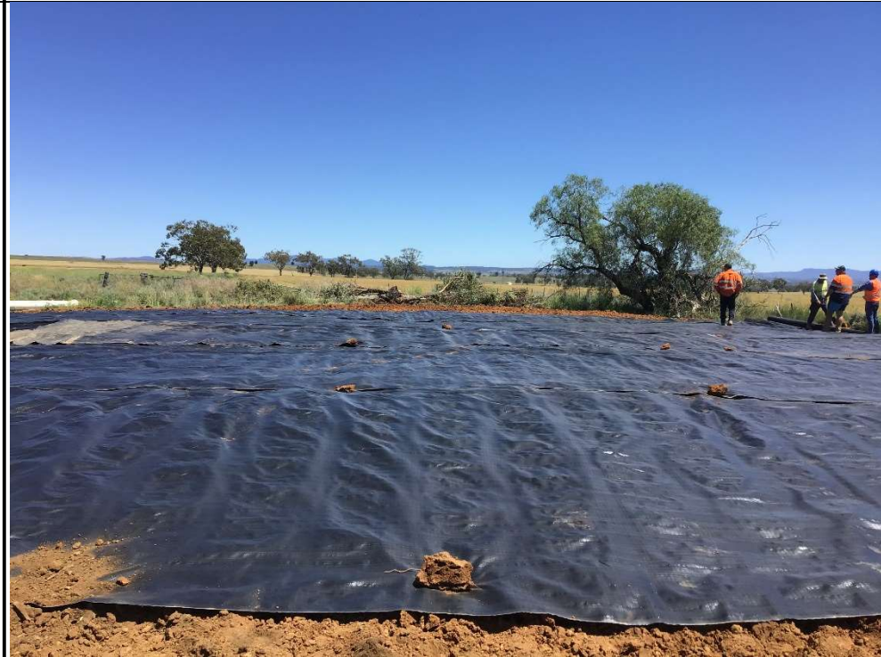
Photograph 26 – High visibility marker layer over Earth Cover Layer, facing west from adjacent TP102
