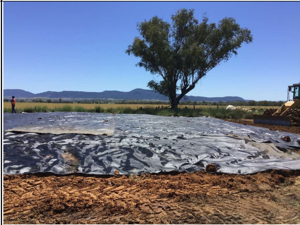
Photograph 25 – High visibility marker layer over Earth Cover Layer, facing north from adjacent TP201
