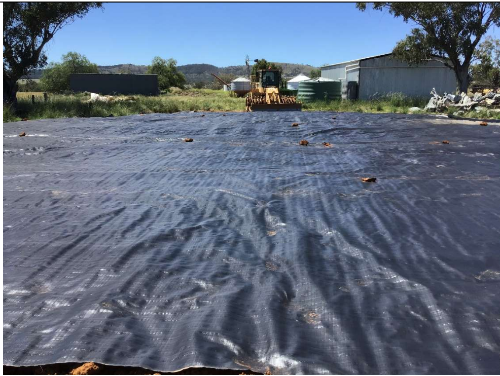
Photograph 27 – High visibility marker layer over Earth Cover Layer, facing east from adjacent TP204
