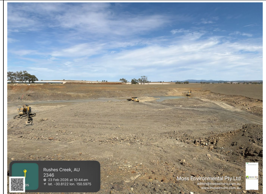
Photo 24 – Ongoing construction activities at the two new dams
