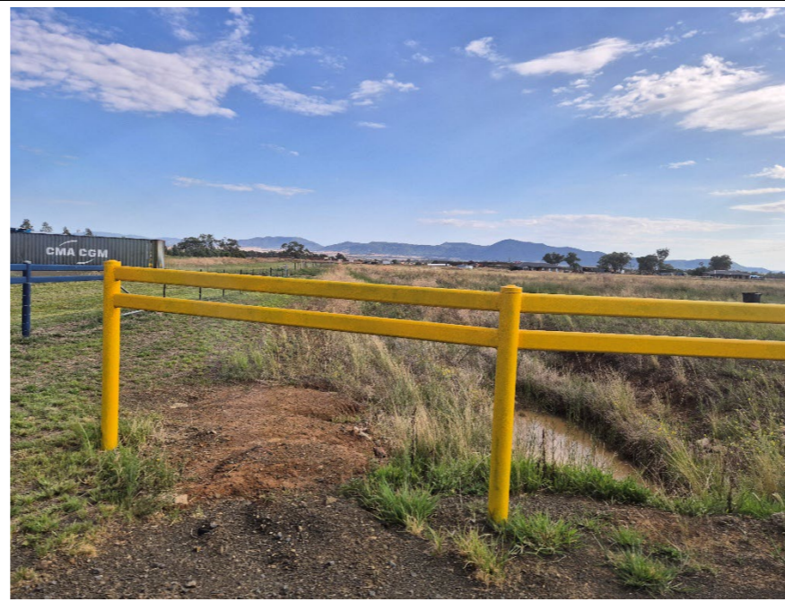
Photo 11 – Clean water diversion trench
