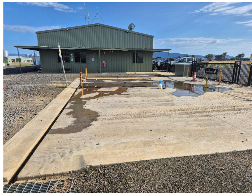
Photo 20 – Wheel wash at entrance
