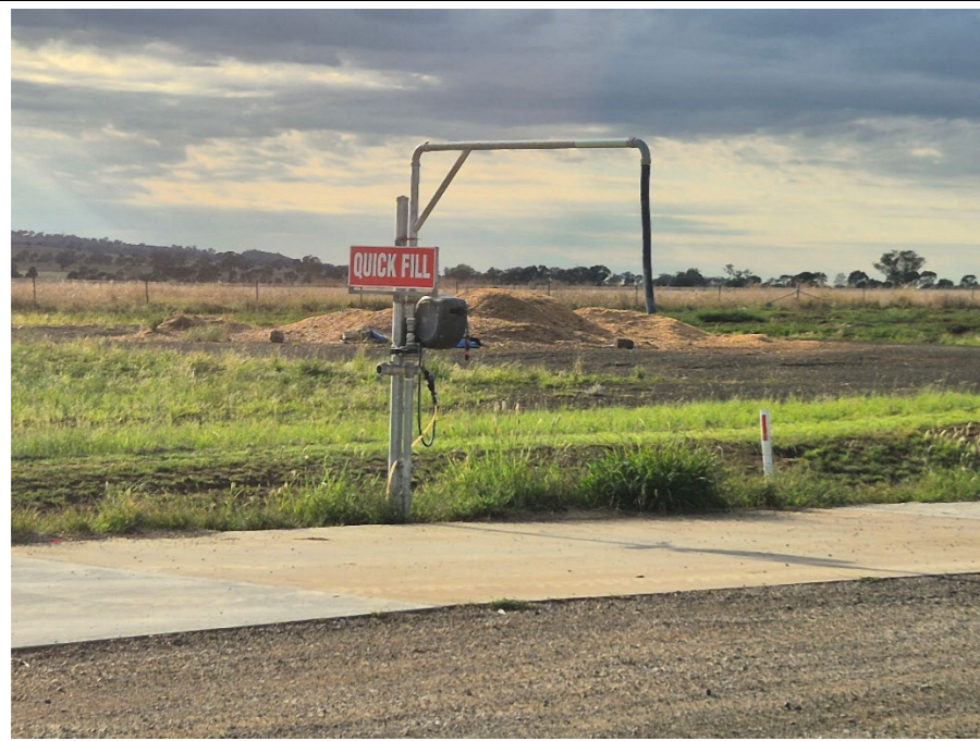
Photo 4 – Dust suppression filling point
