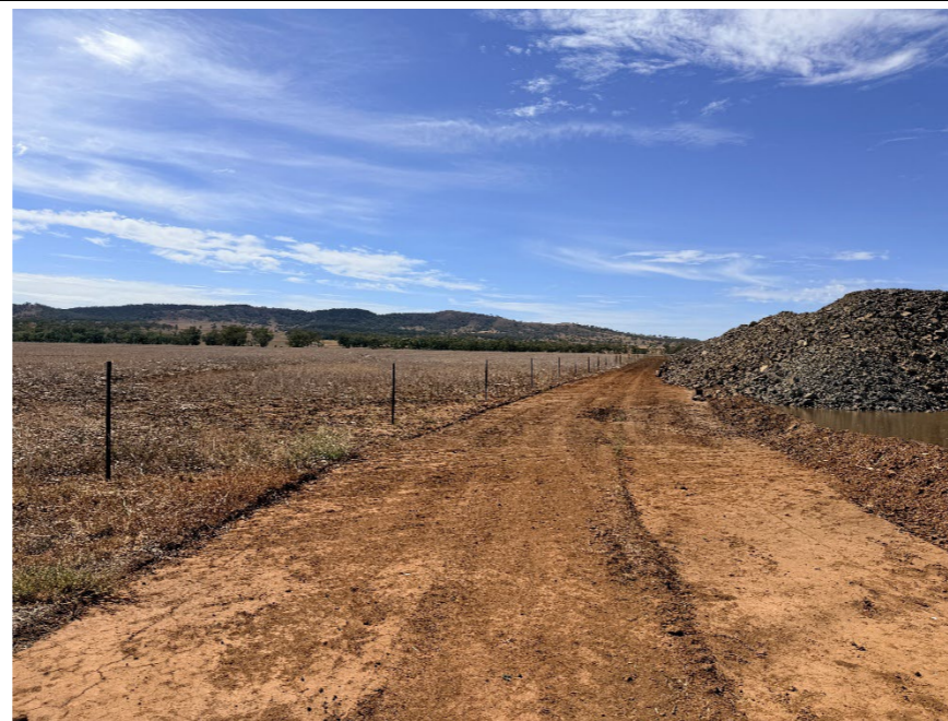
Photo 23 – Sediment fence covered by spoil material
