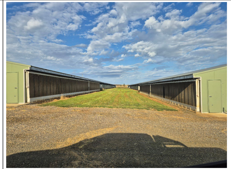
Photo 12 – Grassed swale drains
