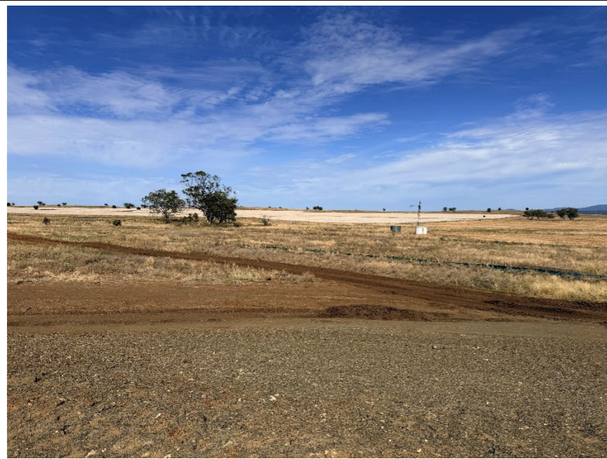
Photo 22 – ErSed controls at two new dams
