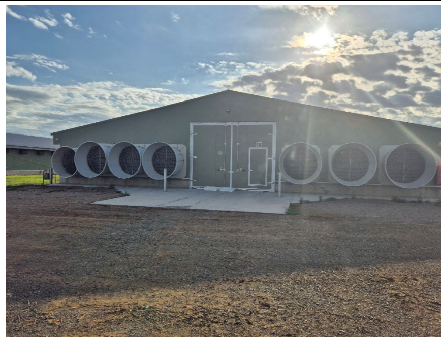
Photo 8 – Vents and fans at the sheds
