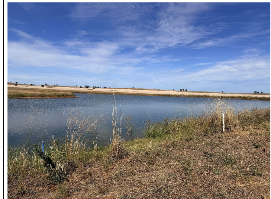
Photo 21 – Overflow pegs at existing detention basin
